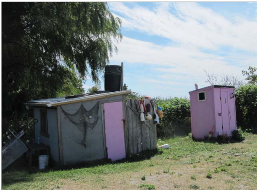
Fig. 95: The outbuildings of Cottage 26 retain some of the historical maritime character of sheds and other small structures along Crab Alley.
