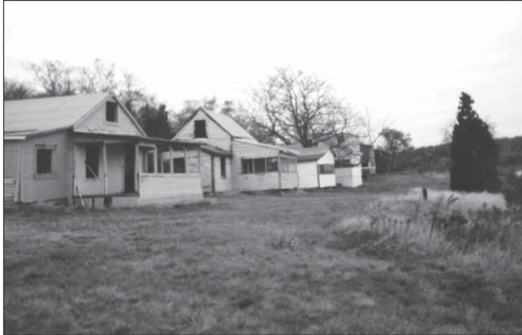
Fig. 91: Cottages 4 and 5 stand empty and awaiting demolition in the 1990s. (Peter Sault)
