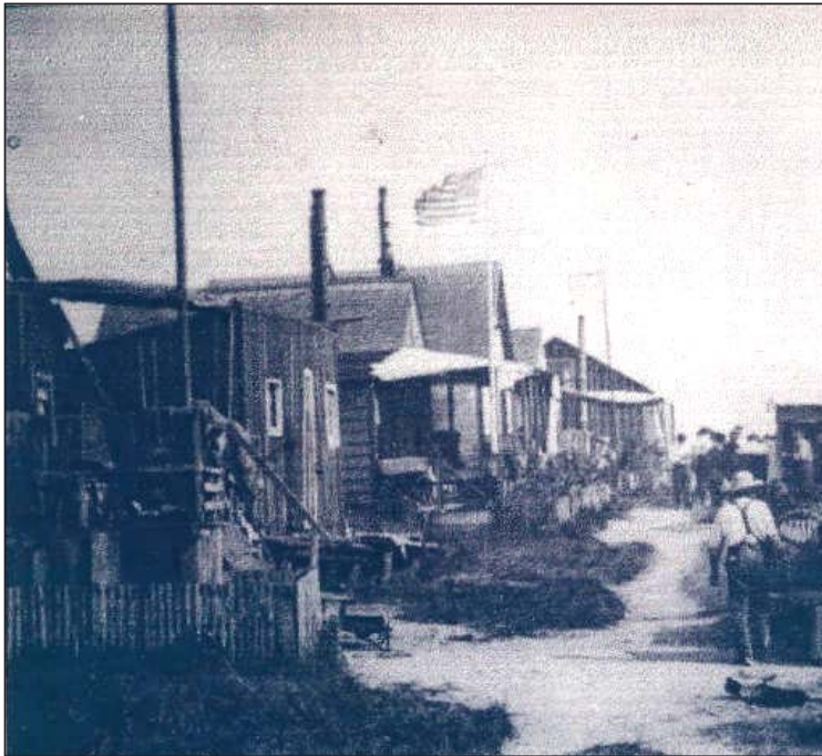
Fig. 33 This undated photo of "Crab Alley" along the southwest-facing side of Middle Head shows a number of people, most or all of them men, working around the toolsheds that lined the shore between the cottages and the sheltered tidal pond that they faced. (Lilian Perry, from collection of Mike McDevitt)
